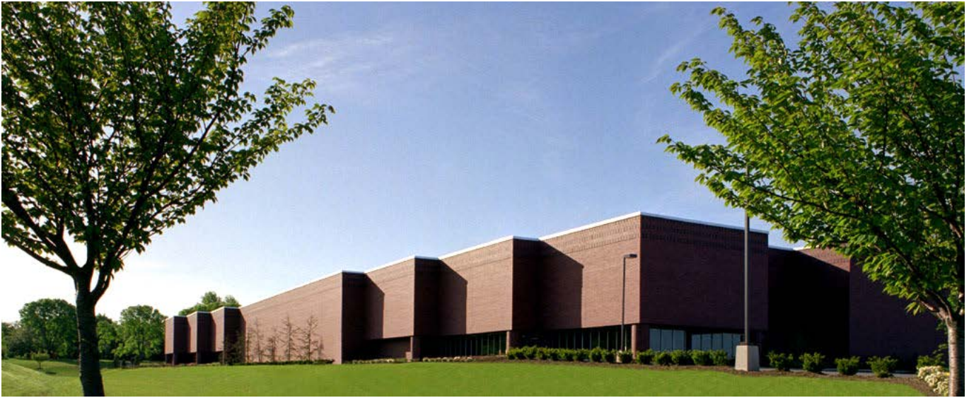
Forsgate Warehouse, South Brunswick, NJ
