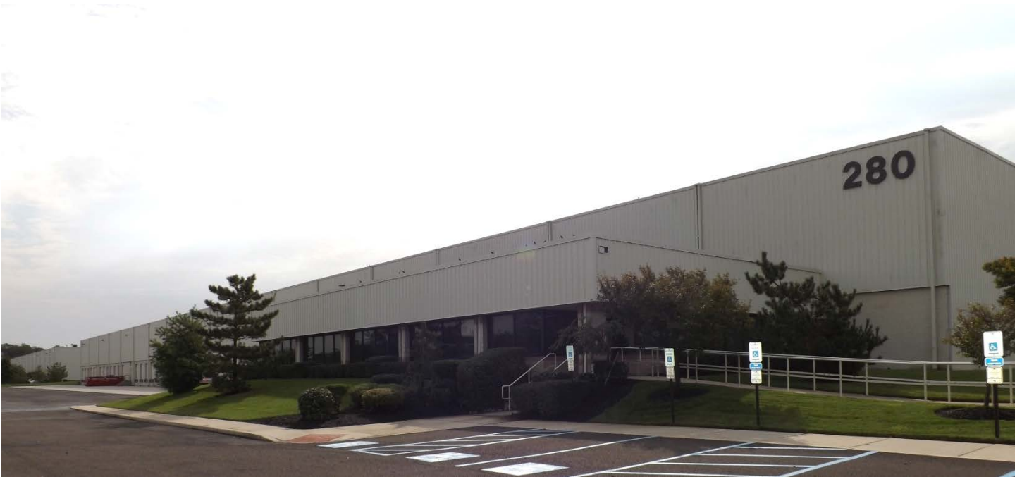
Whitesell Warehouse, Florence, NJ
